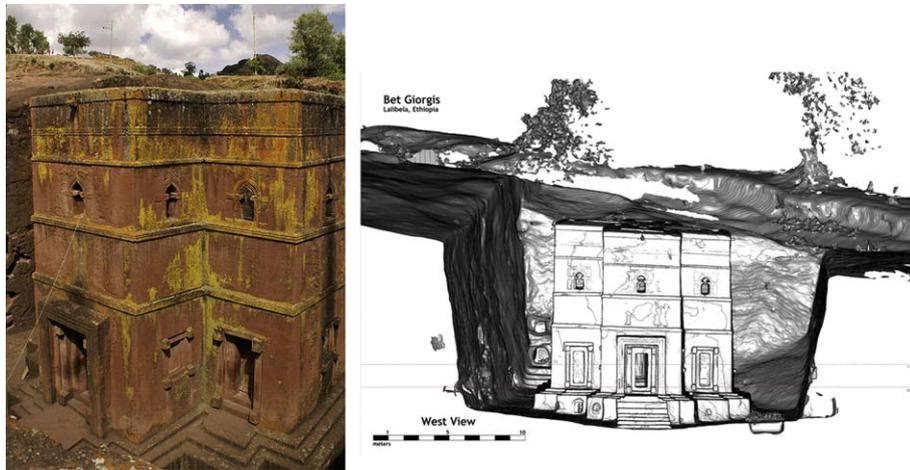
**Fig. 3.** Bet Giorgis Church, Lalibela, Ethiopia – 12th century AD rock-hewn Coptic church. Left – photograph of the church facade; Right – west facade view of the church derived from laser scan demonstrating this extremely useful by-product of scanning.
